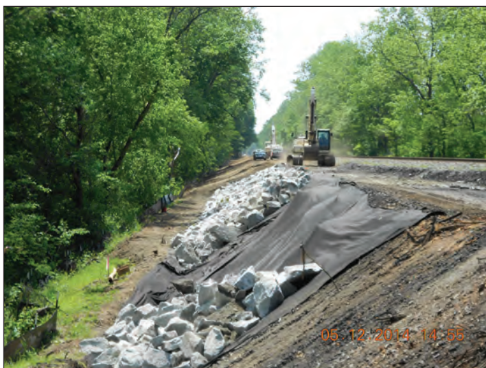
C-4901 Bowers to Lake - embankment stabilization
